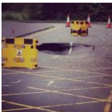
Sink hole opens up near Kassam Stadium
