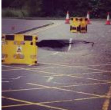
Sink hole opens up near Kassam Stadium
