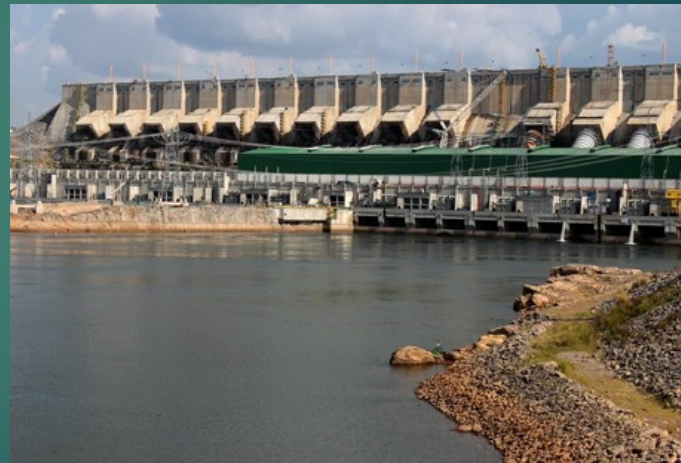
Belo Monte (Main turbines)
